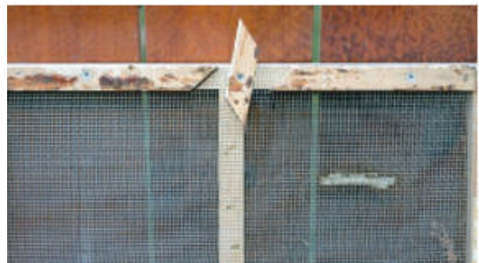
Figure 4 Double screen entrance in the open position
